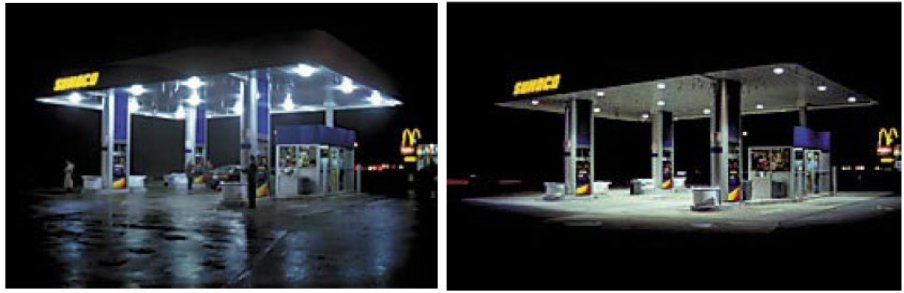
The above photographs illustrate the impact of glare on a lighting installation. The left photo has high-glare, non-recessed fixtures under the canopy. Note how bright the lights themselves are and how dark the pump area is. The right photo shows the same gas station canopy with full-cutoff, recessed fixtures. Note how the light is directed effectively toward the gas pumps. Images from http://www.skyandtelescope.com
